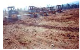
Houses and farms are bulldozed in Aung Ra village
