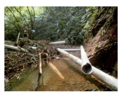
Photo: Water supply pipe washed away by stream flood in Maliyang relocation camp on September 19, 2012.
