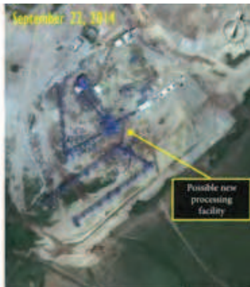
fig 4: Between May 14 and September 22, 2014 imagery shows infrastructure was erected in the southern portion of the area analyzed. The new structures appear to be a possible processing facility for the mine.
