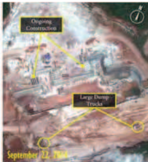
fig 3: Ongoing construction can be seen in imagery from September 22, 2014. Additional foundation footings are present along with large loaded dump trucks. The function of the large structure cannot be determined at this phase in construction.
