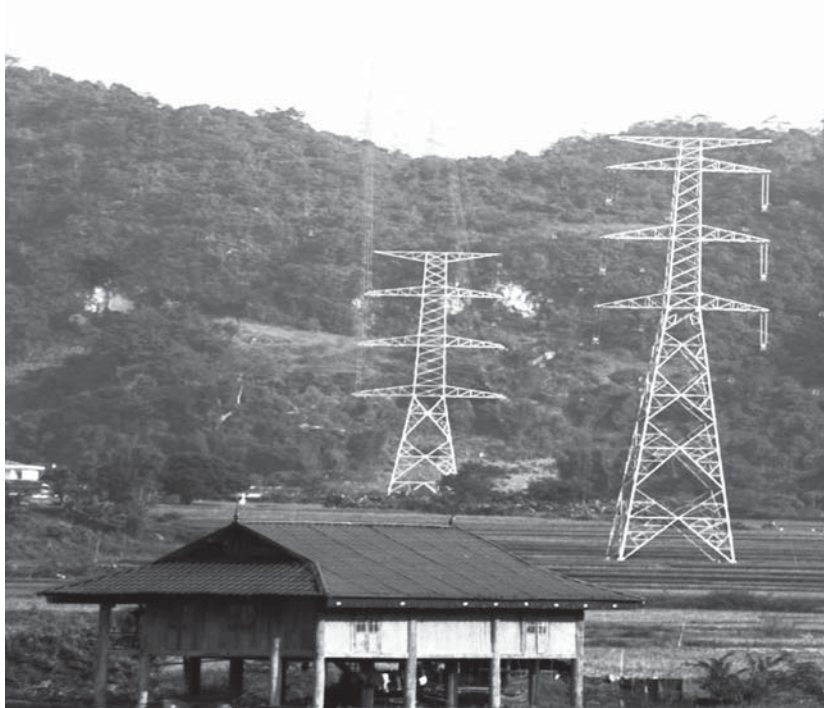
The transmission line across the Ta Niet Village, Chieng Hac Commune
