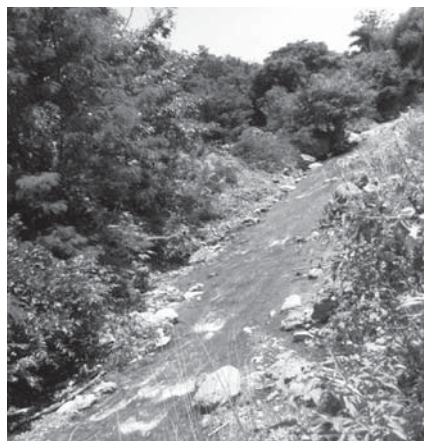
photo of new drain made by irrigation officer
