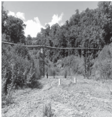
photo of useless new drain
