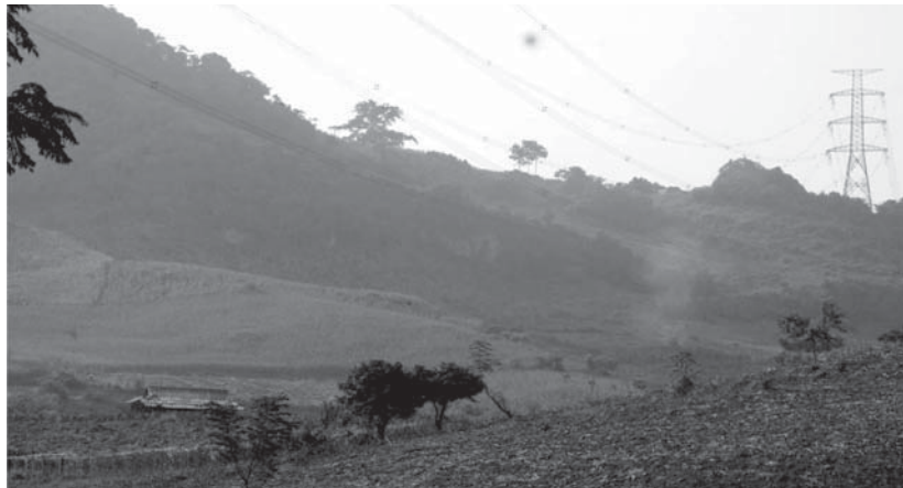
Mr. Son Nguyen Van's house (Ta Niet Village, Chieng Hac Commune) is still under the transmission line
