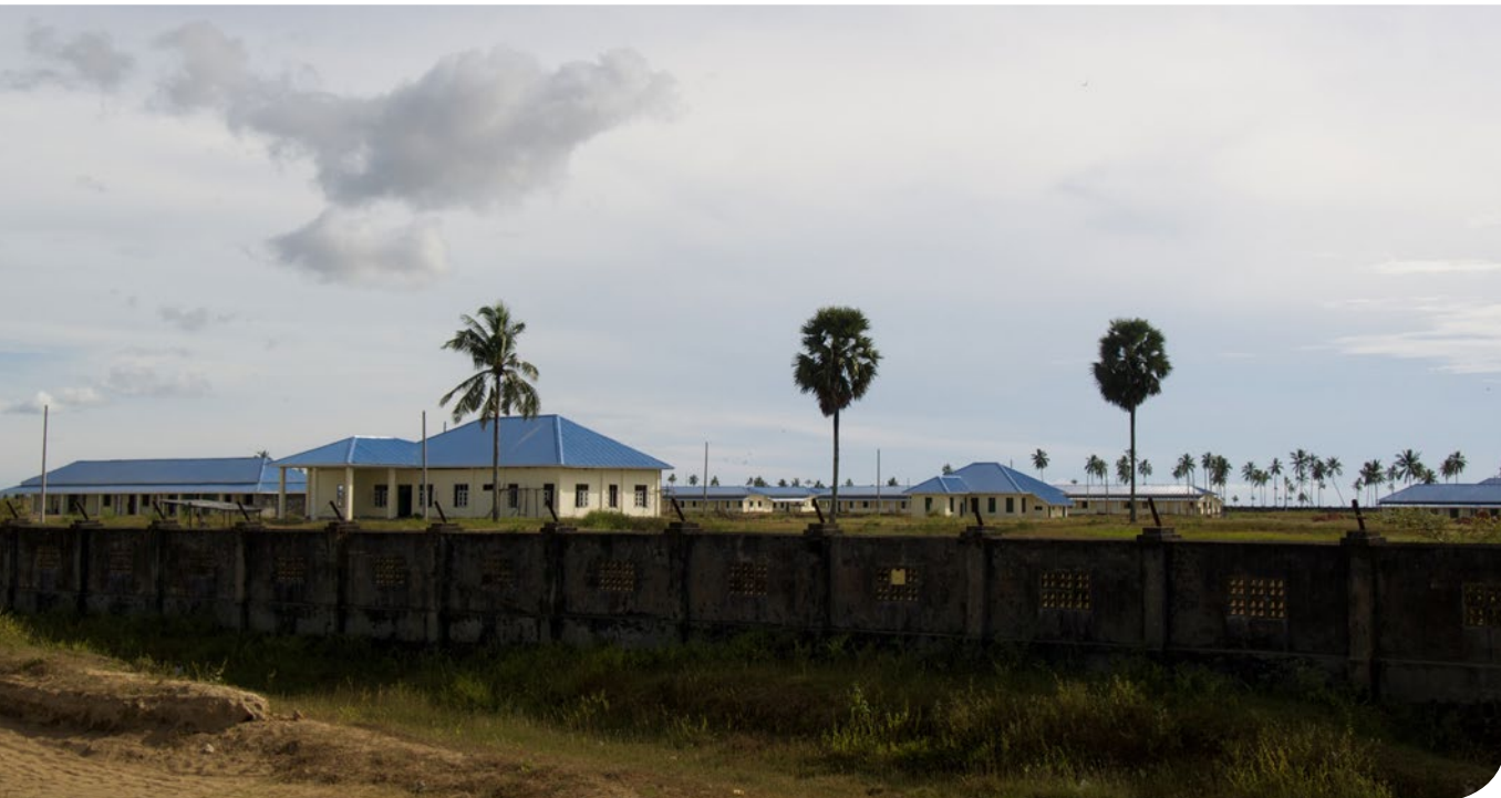
Police buildings under construction adjacent to Rohingya detention camp complex, Sittwe, December 2014
