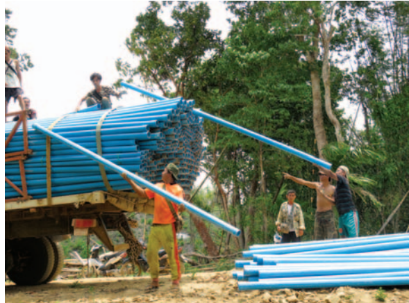
PVC pipes being delivered to Washuko village
