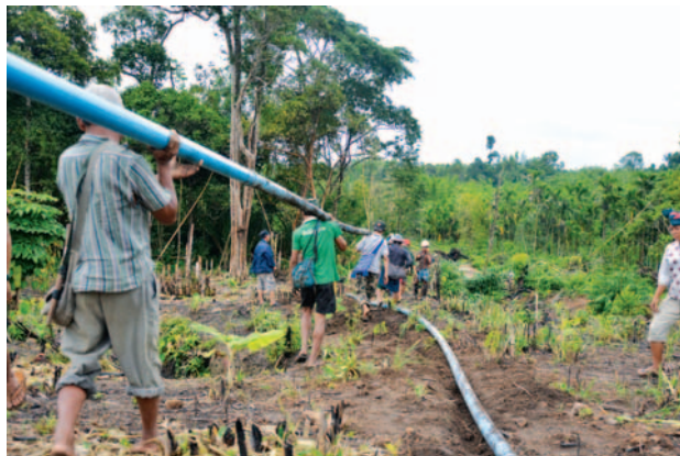
Volunteers from the village work together to bury the water pipe system
