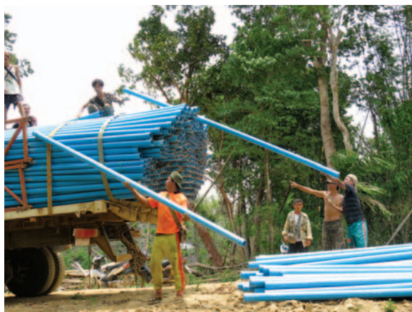
PVC pipes being delivered to Washuko village
